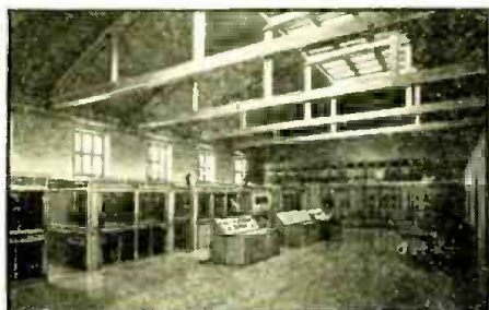
The transmitter room of the new high-power broadcast station in Finland.
